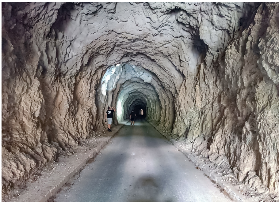
Figure 1. The interior of the tunnel at the mouth of the Lim river.
